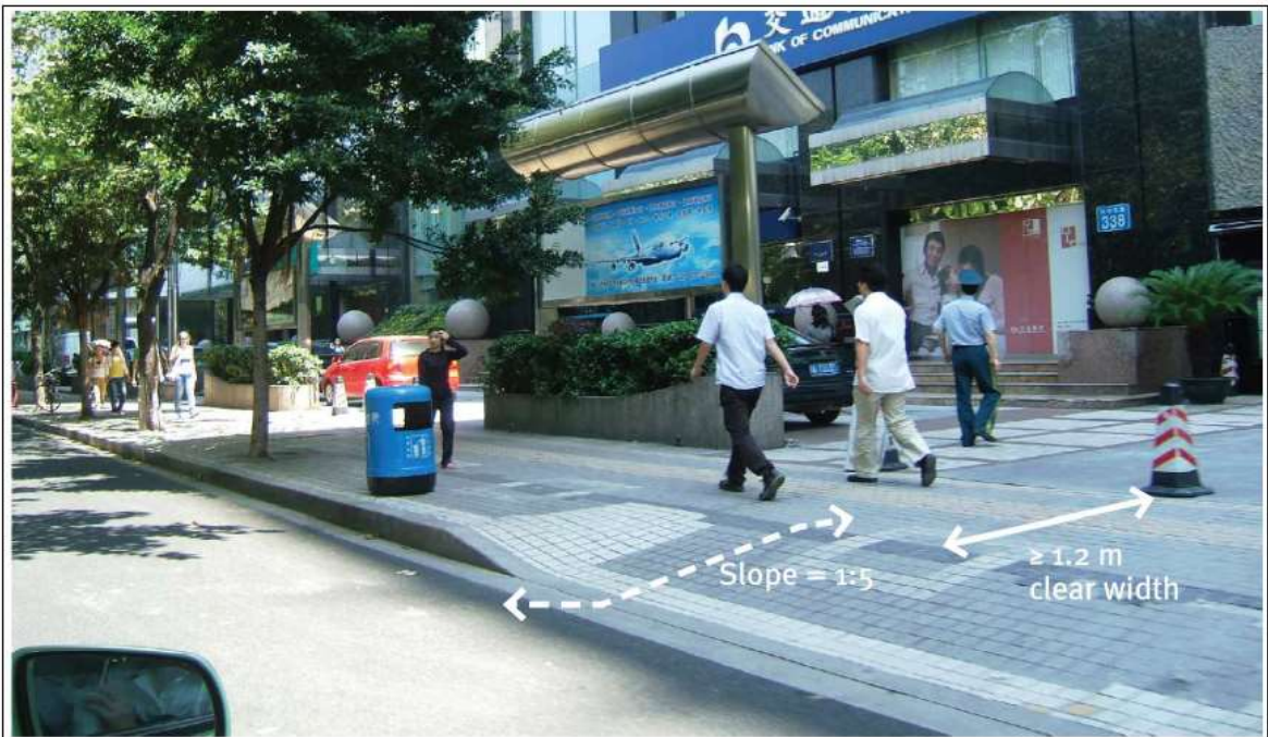
CONSTRUCTION OF FOOTPATHS AT PROPERTY ENTRANCES
